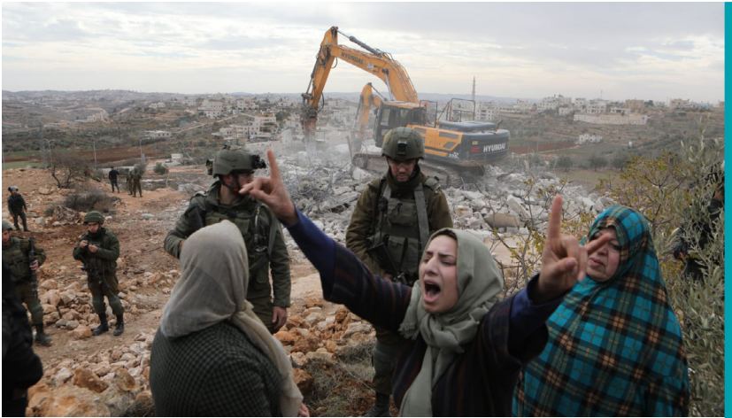
During the demolition of Palestinian homes by the occupation forces in Masaf-er Yatta - Hebron. Picture by Ma'moun Wazwa
