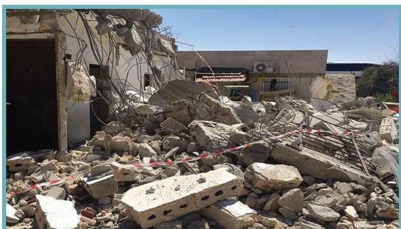
A self-demolished house that belongs to M. family in Jabl Al-Mukabber. July 25, 2021.
