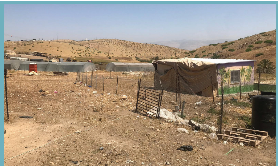
A school was demolished more than once by the Israeli forces in Al-Maleh-Tubas, the Northern Jordan Valley. The school was rebuilt again after multiple demolitions. May 28, 2021
